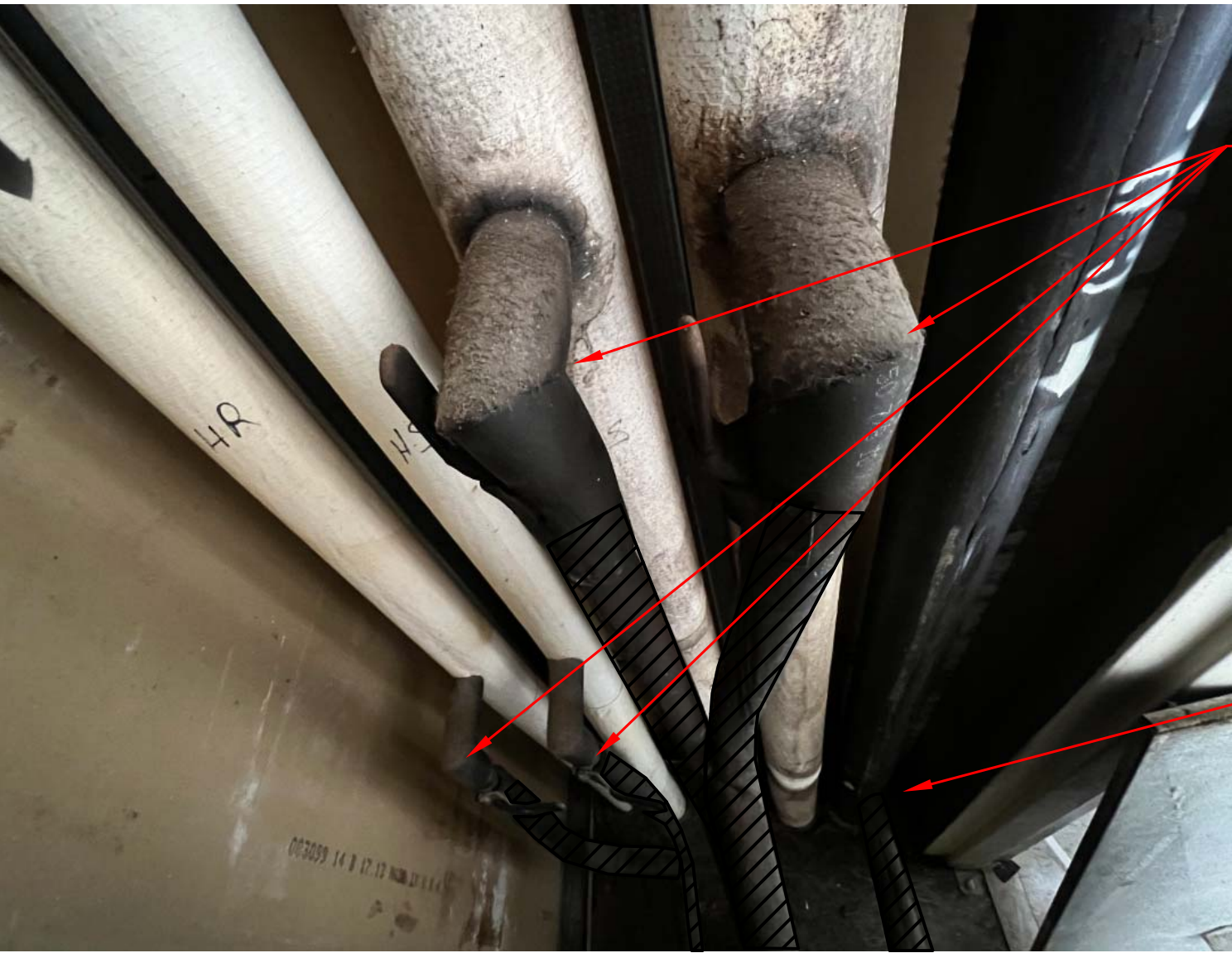
3 EXISTING PIPING RISER & CONNECTIONS TO COILS (TYPICAL) SCALE: NTS
