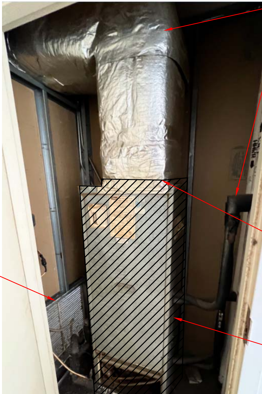
1 EXISTING FAN COIL UNIT (TYPICAL) SCALE: NTS
