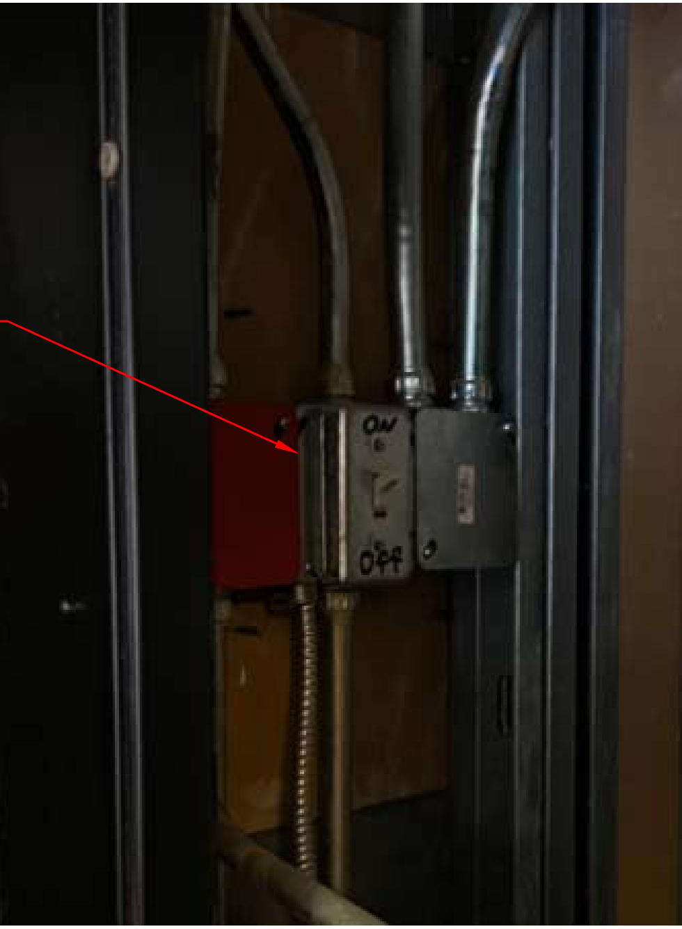
5 EXISTING DISCONNECT SWITCH (TYPICAL) SCALE: NTS
