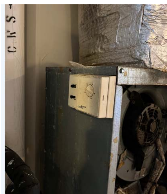
4 CORRIDOR FCU THERMOSTAT (TYPICAL) SCALE: NTS
