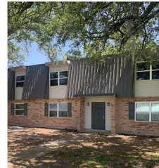
RENAISSANCE OAKS HOUMA IN CONSTRUCTION
