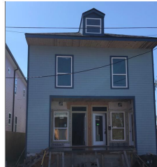
NORA St. ANN, NEW ORLEANS IN CONSTRUCTION
