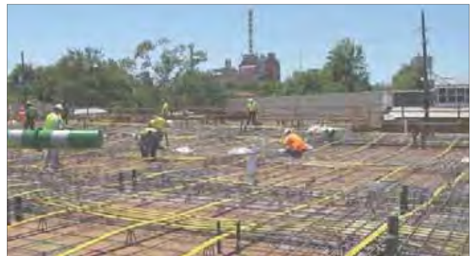
Current Construction Progress
