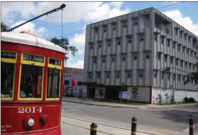
Existing Building Photos
